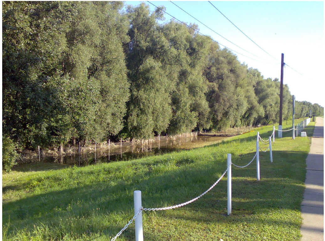
figure 20 Row of trees in front on the dike to reduce damage from ice (Bognar Zoltan, OVF, Hungary).
